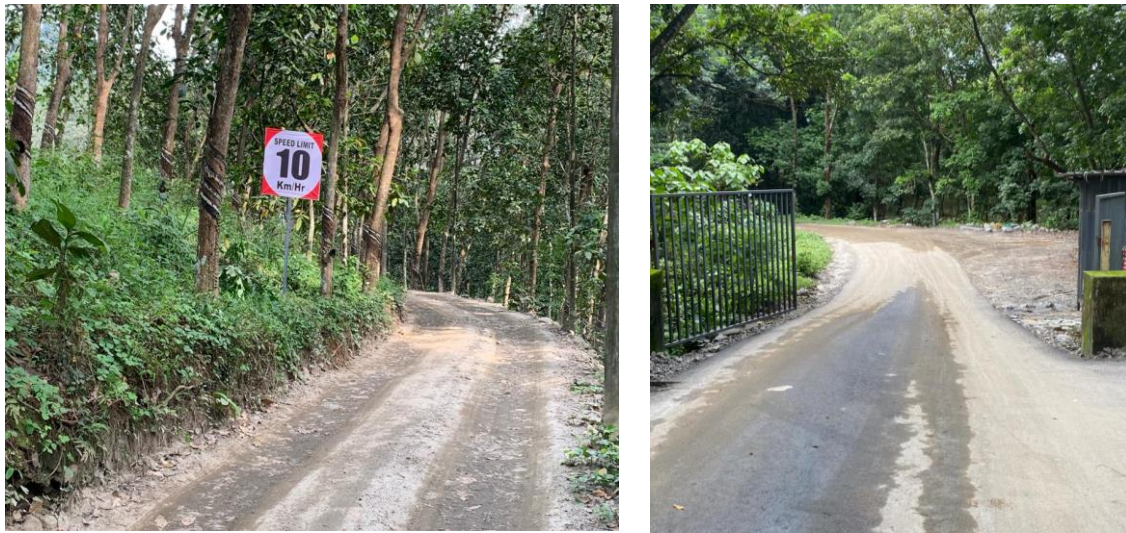
Figure 5: Photograph of Access Road to Quarry
